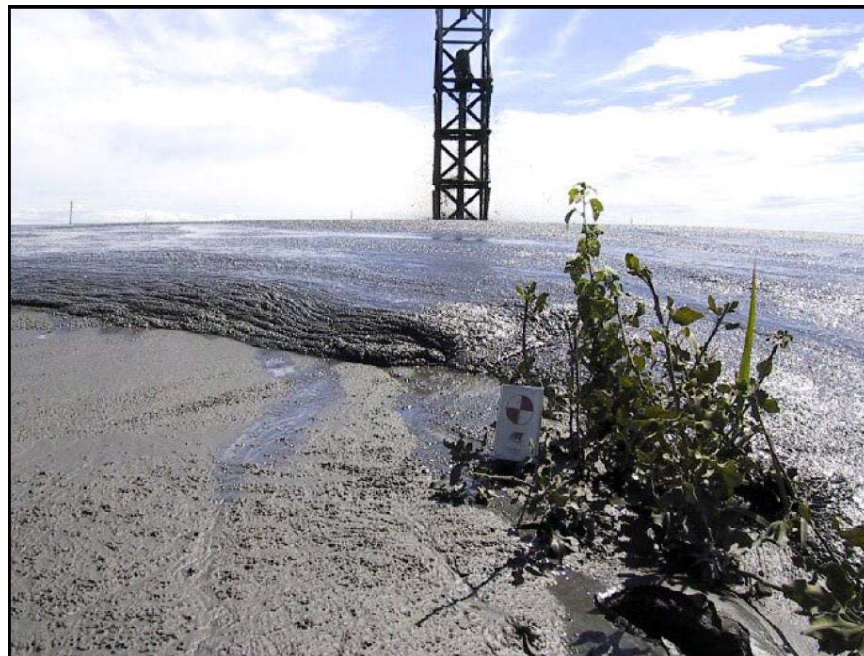
Figure 2 Photograph of a thickened tailings disposal (TTD) system ( http://www.tailsafe.com/photos/partner_paste-technolgy/03-06-12_paste-technolgy_pa.gif ).
