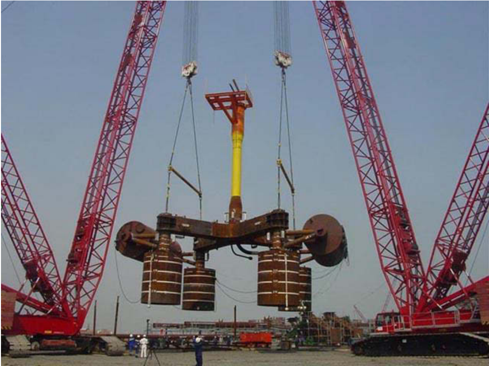
Figure 1-13. Side view of caissons ( www.noed.com.cn )
