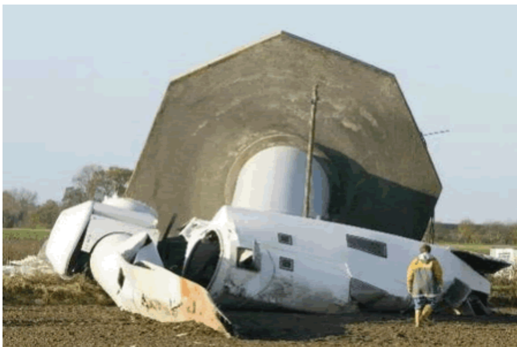
Figure 1-8. Failure of a wind turbine due to overturing of the structure (photo courtesy of Con-tech system Ltd)
