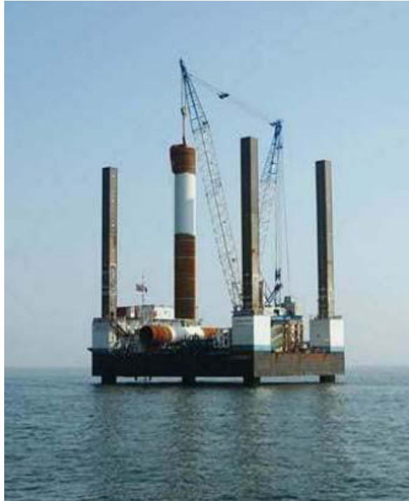
Figure 1-11. Installation of a monopile for an offshore wind turbine ( www.hornsrev.dk )
