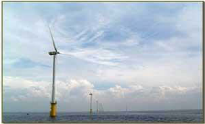
Figure 2-1. Egmond aan zee wind farm located in the North Sea ( www.trelleborg.com )
