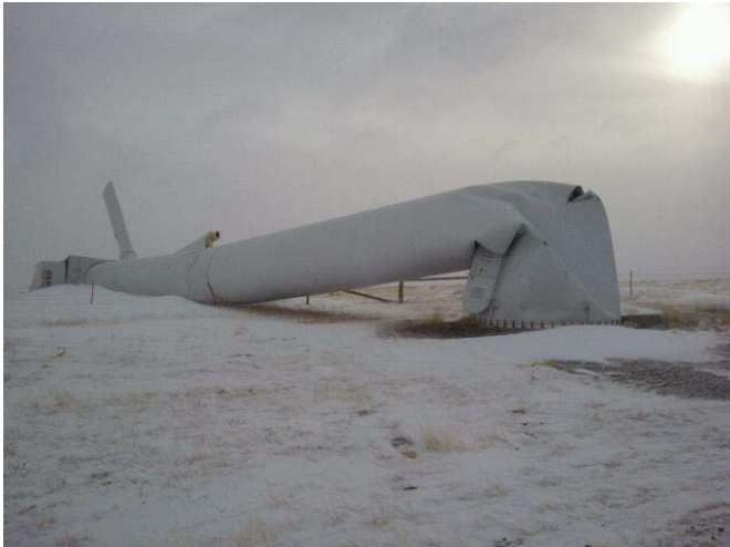
Figure 1-6. Failure of a wind turbine’s tower in Wyoming, 1/Feb/2011 (Photo courtesy of Eric Nielsen)
