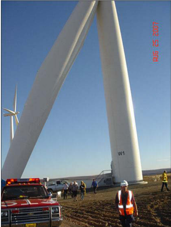
Figure 1-5. Failure of a wind turbine in respect to the bending moments acting on the tower (Photo courtesy of Brian Hulke)
