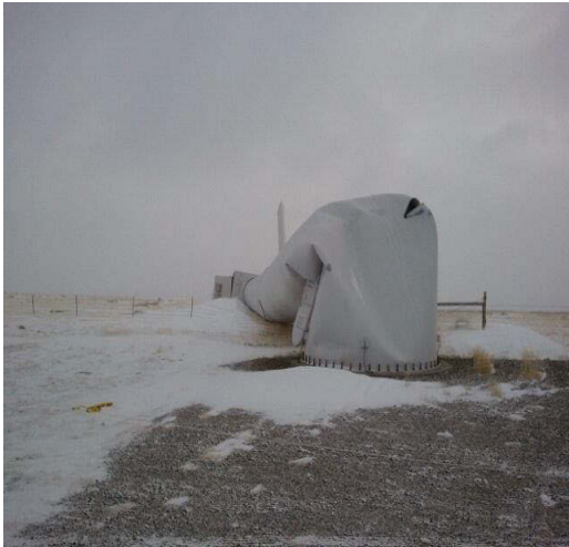
Figure 1-6. Failure of a wind turbine’s tower in Wyoming, 1/Feb/2011 (Photo courtesy of Eric Nielsen)
