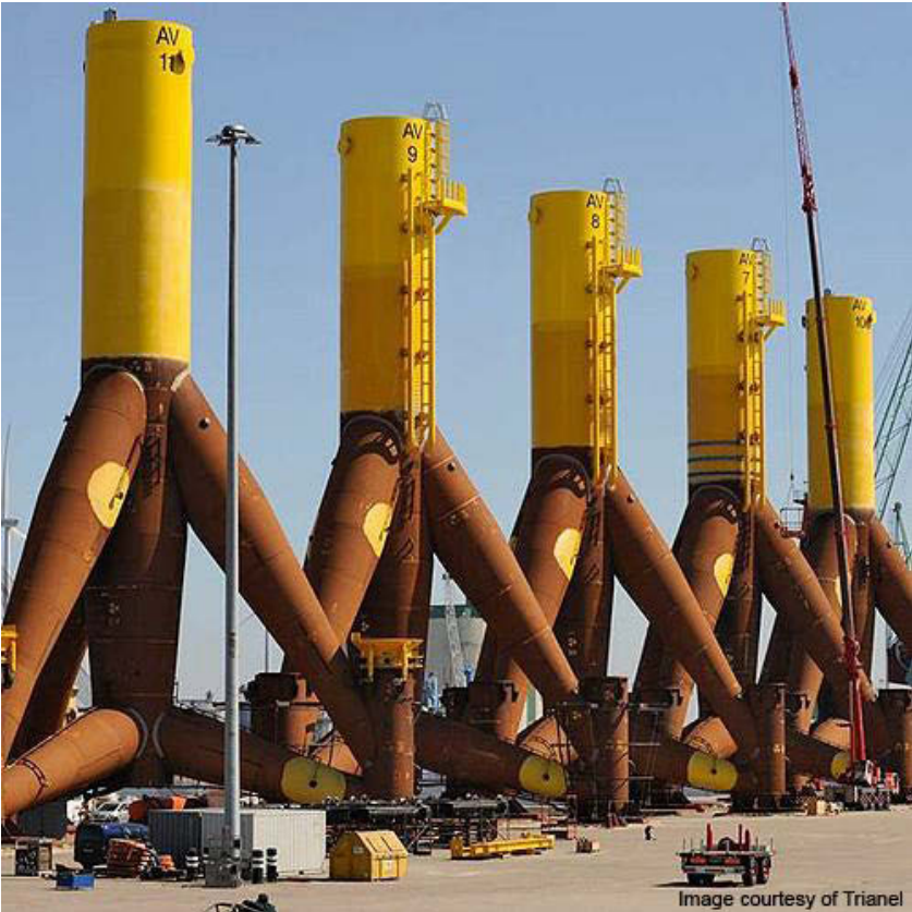
Figure 1-14. Tripods used for offshore wind turbines (Photo courtesy of Trianel Ltd)
