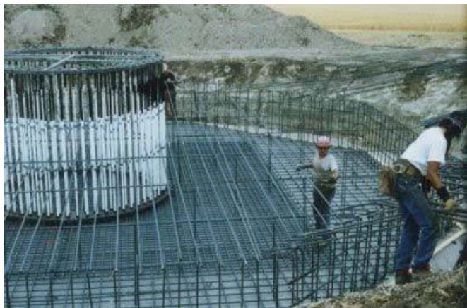
Figure 1-12. An onshore raft foundation for a wind turbine during construction ( www.johnrsweet.com )
