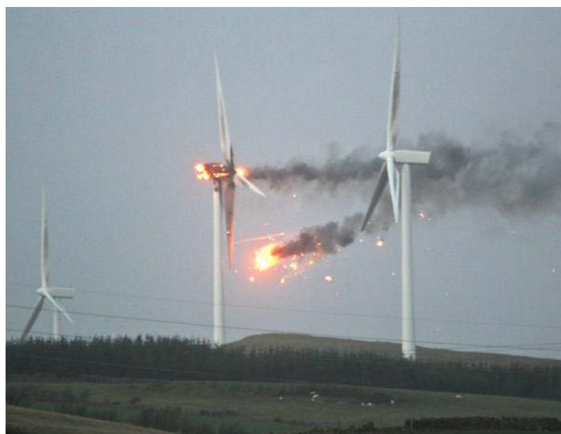
Figure 1-4. Failure of a wind turbine associated with electrical problems (Photo courtesy of Stuart McMahan, adopted from www.newscientist.com )
