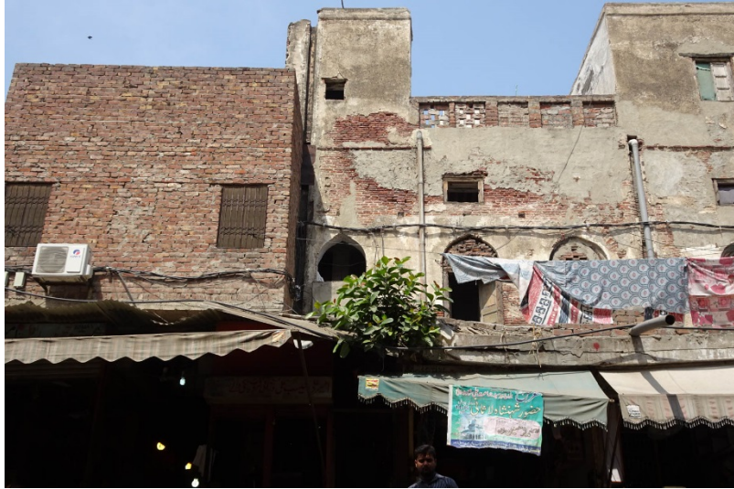
Figure 1. Split air conditioner fitted to uninsulated brick building in Lahore (2016: outdoor unit can be seen at far left side)
