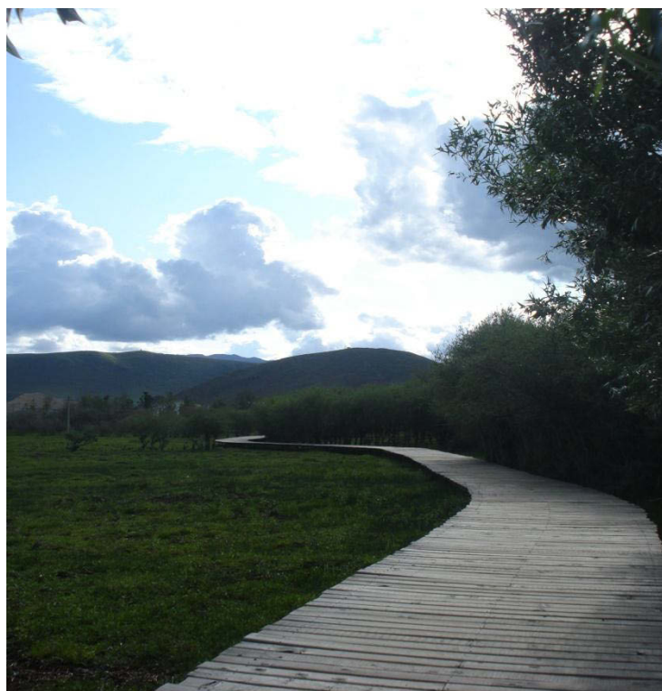
Photo 10: A raised walkway built around the lake in front of Songtsen Ling Monastery for both pilgrims and tourists to circumambulate without damaging the wetland.
