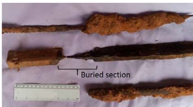
88 89 Figure 1: Corroded reinforcement from 30-year-old CSRE wall
