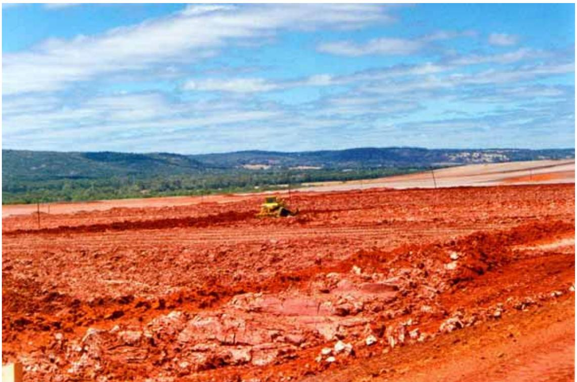
*Plate 2.3. Bulldozers cultivate the surface to assist in drying of the residue layers. However, excessive heavy vehicle traffic can cause sub-surface compaction. Crystallisation of dissolved salts is often seen on the surface of recently-dried residue.*
