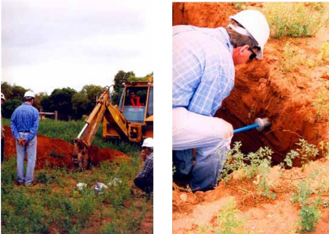
**Plate 7.2.** Digging machinery assisted in access to the profile for taking soil cores and insertion of TDR probes.
