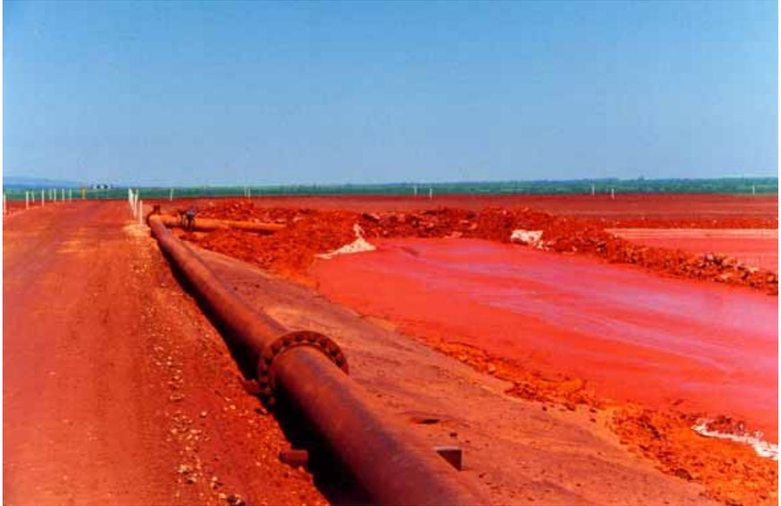
*Plate 2.2. Bauxite residue sand and red mud is pumped and spread across the residue impoundments at Pinjarra.*
