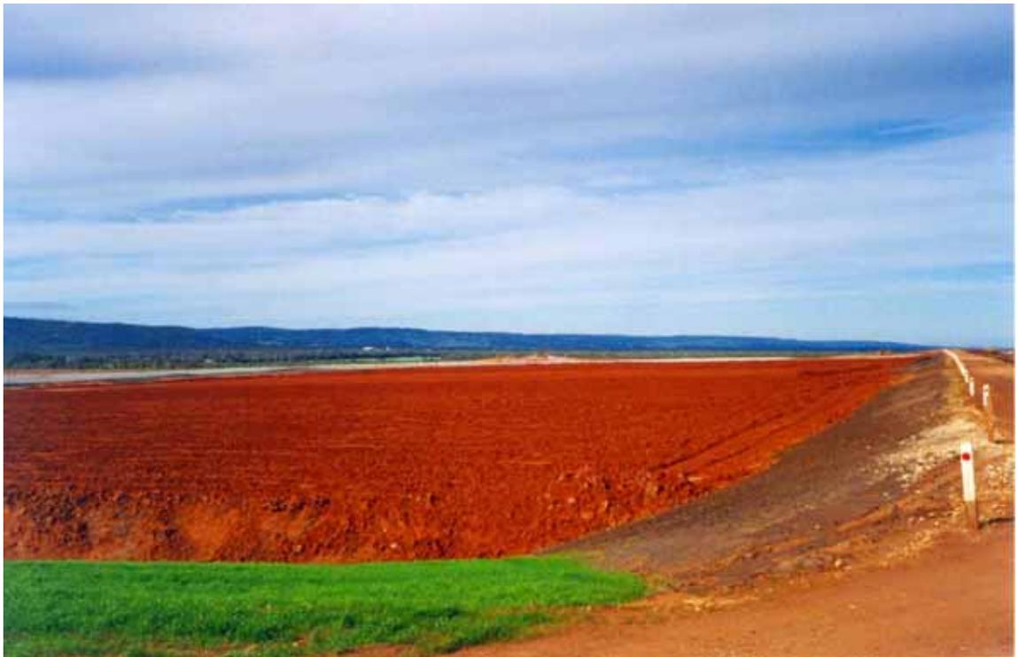
*Plate 2.1. Bauxite residue dries within impoundments by air exposure assisted by surface cultivation.*
