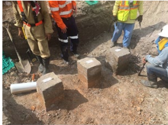
Figure 4. Excavated block samples at one test site location.
