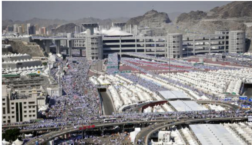
Figure 2-2: Aljamarat Bridge. Source: Edrees (2016).
