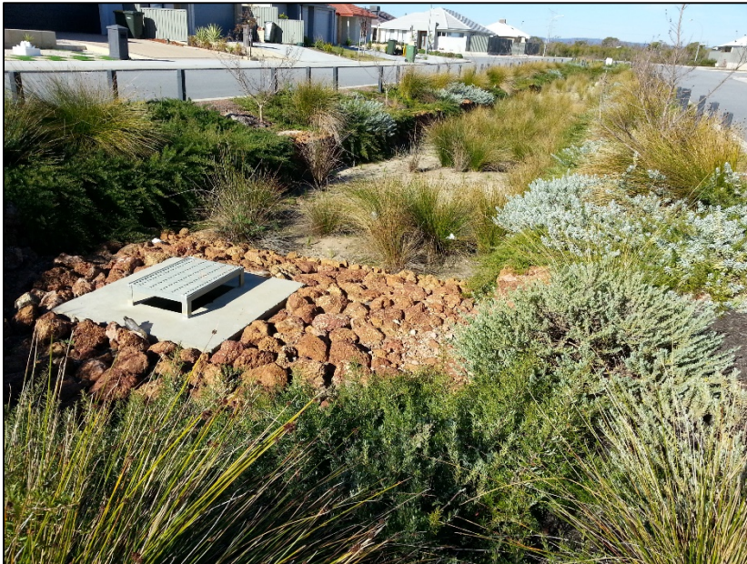
Figure 3: An example of a 'living swale' in a median strip This 'living swale' constructed and vegetated as a strip in the centre of a road in a new residential development allows for the retention of stormwater on-site, and slow infiltration. Image credit: Leah Beesley
